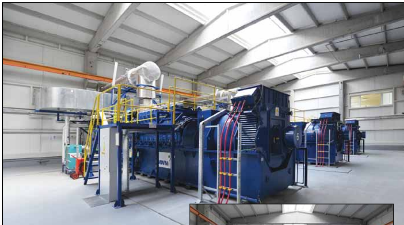
Tekno Energy's Bilecik power station can produce a total output of 26 MWe using six TCG 2032 V16 engines by MWM.
