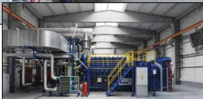
Tekno Energy's Bilecik power station can produce a total output of 26 MWe using six TCG 2032 V16 engines by MWM.
