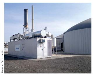
Since it was installed, the biogas plant at Löberitz has also served as a test plant for the process technology used by MWM. Components are tested under real conditions and measurements taken. At the moment, catalytic converter trials are being run for two research projects and a catalytic converter manufacturer. These projects are implemented by MWM in collaboration with the German Biomass Research Centre.
