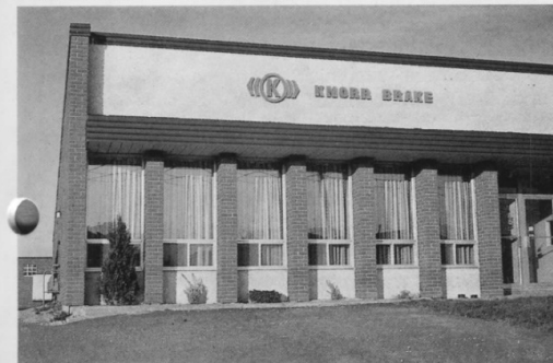
Knorr Brake Limited, Mississauga
